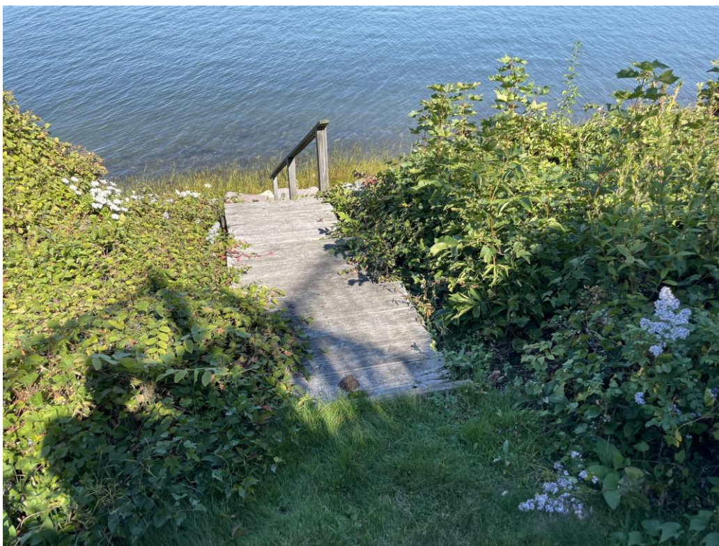
Photograph #6 – View of the existing stairway.
