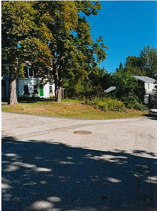
Photograph 1. – Front of dwelling, 214 Hull Street, Hingham,
