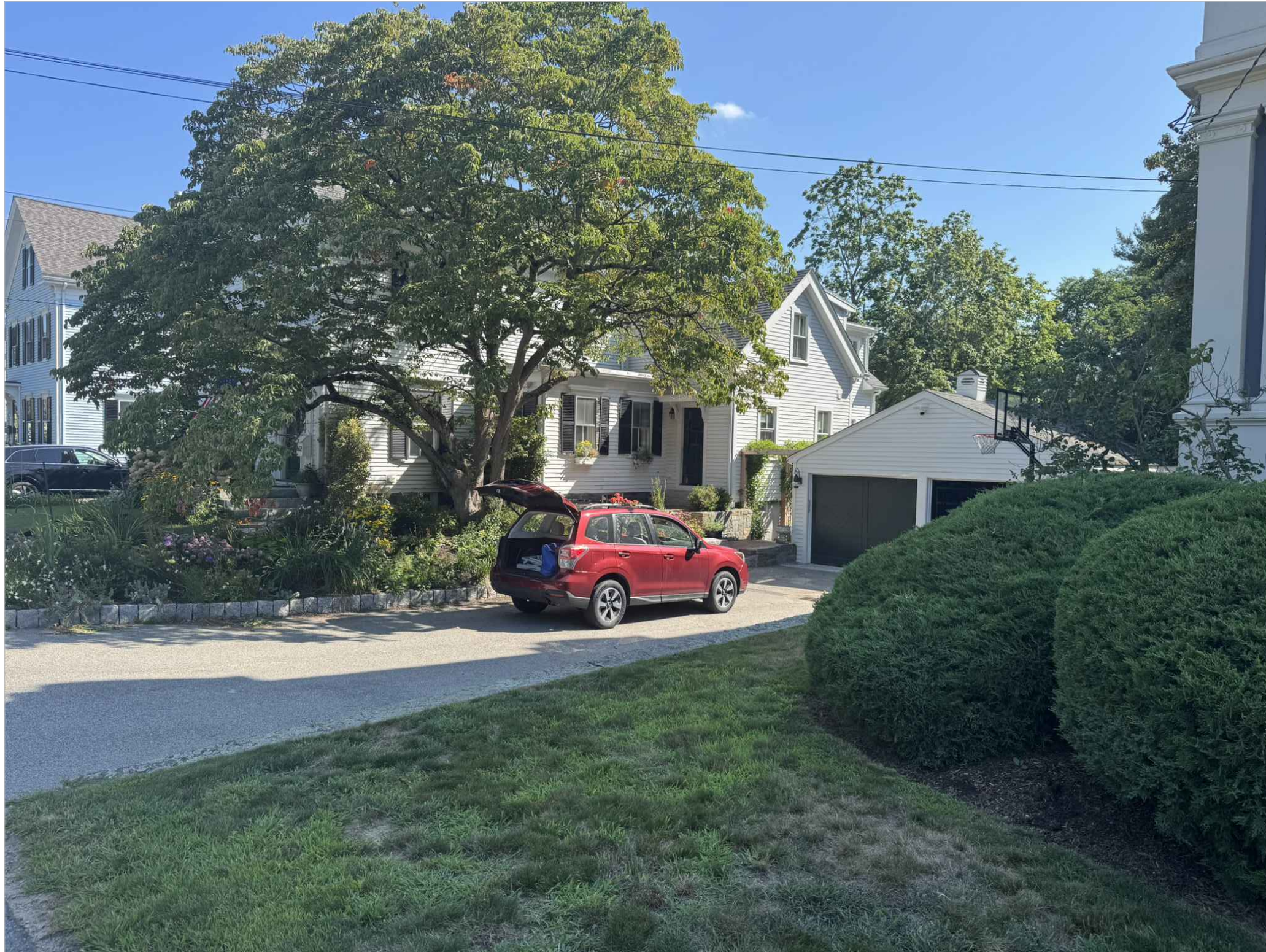
PHOTO EXHIBIT 2 - EXISTING SOUTH ELEVATION
