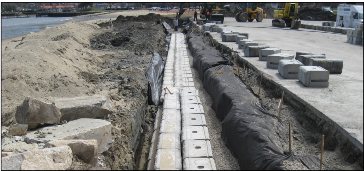
Figure 5: Dune core placed as an early attempt to stabilize the later constructed coastal dune
