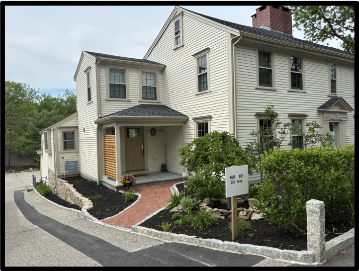
FRONT FACING NORTHEAST
