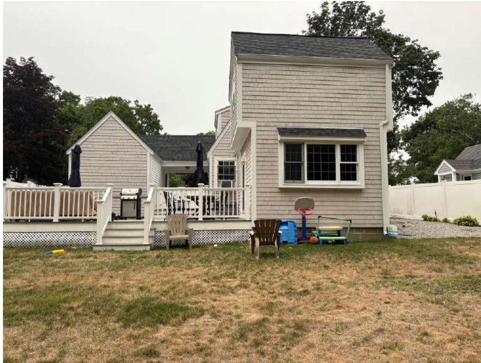
Photograph #3 – View of the back of the single-family home and proposed addition location to the right.
