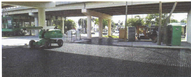
FLODOT Underpass Project
