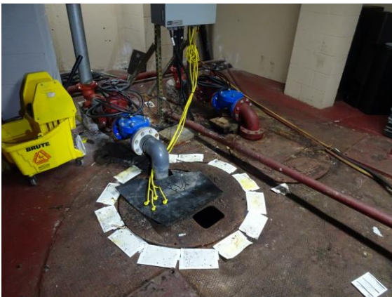
Sanitary ejector system.
