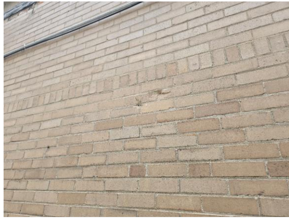
Spalled brick.
