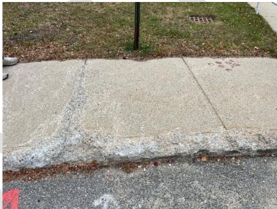
Damage to concrete sidewalk and curbing from snow removal and freeze/thaw cycling.
