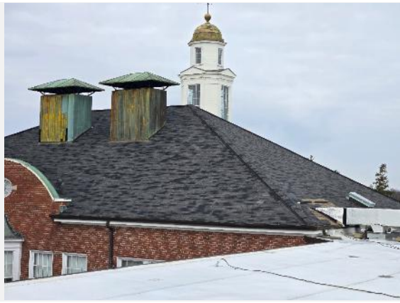
Asphalt shingled roof.
