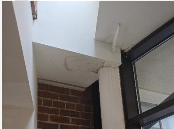
Stained ceiling below skylight and metal roof at courtyard.
