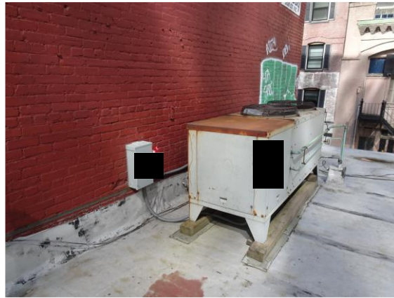
Typical HVAC split system condensing unit.
