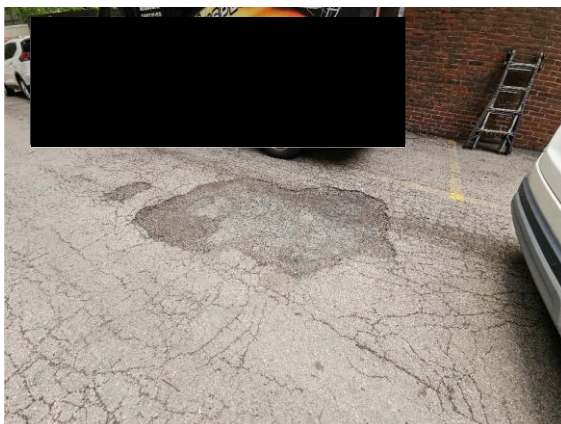
Asphalt driveway at loading dock.
