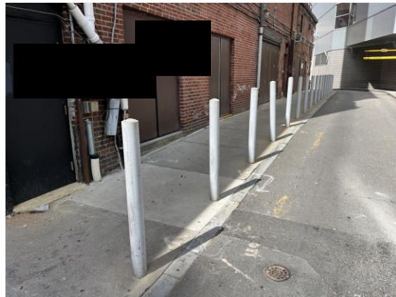
Alley along the north elevation of the building.
