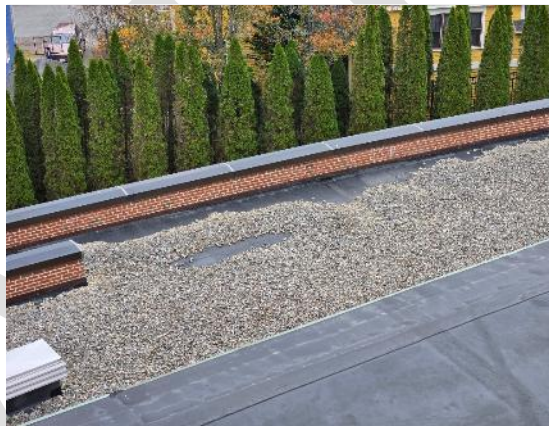
Ballasted EPDM membrane roofing.
