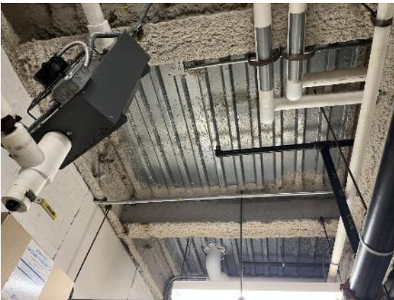
Steel and corrugated metal decking in 2002 addition.
