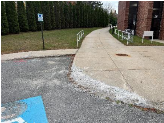
Damage to concrete sidewalk and curbing from snow removal and freeze/thaw cycling.
