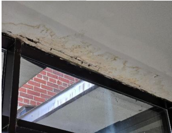
Stained ceiling below skylight and metal roof at courtyard.
