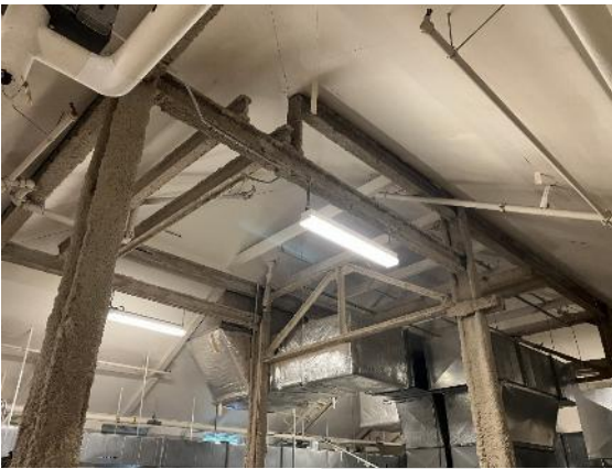
Typical steel framing, load bearing masonry and concrete slab in the 1935 section.
