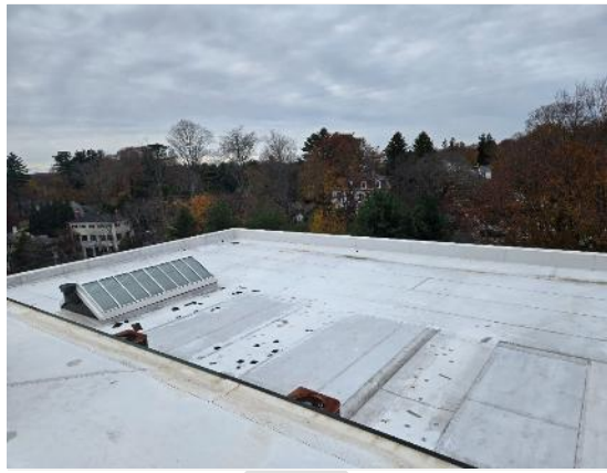
TPO membrane roofing.
