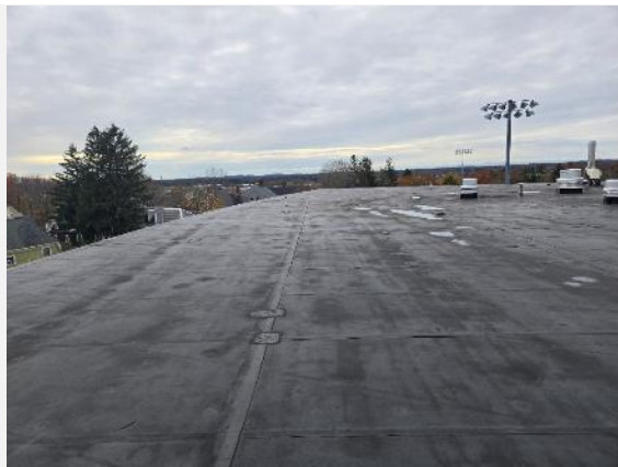
EPDM membrane roofing.
