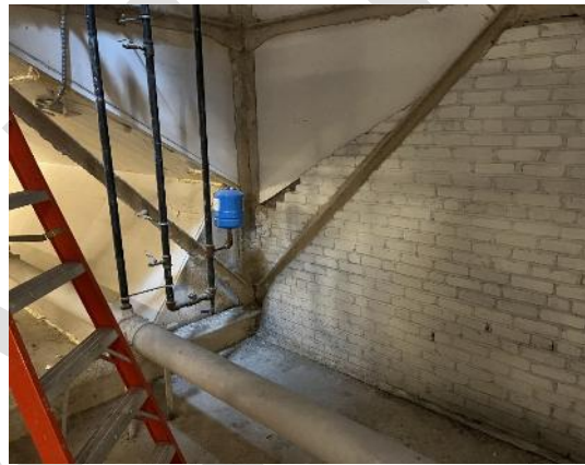
Typical steel framing, load bearing masonry and concrete slab in the 1935 section.
