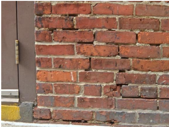
Deteriorated mortar.
