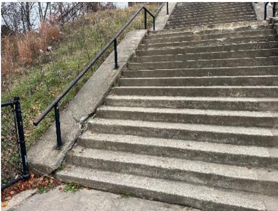
Damage to concrete staircase between football and baseball fields.
