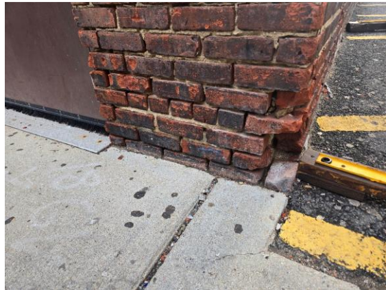
Missing/loose bricks.
