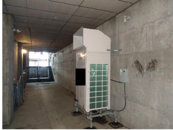
Typical split system condensing unit.
