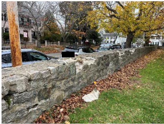
Degraded fieldstone wall along [REDACTED]
