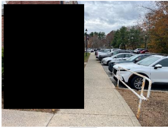
Typical sidewalk around building.
