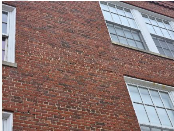
Step cracking.
