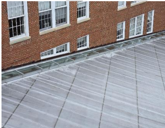
Metal roofing and skylight.
