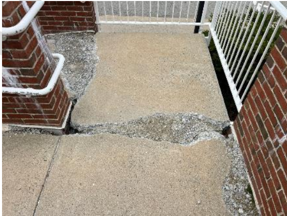
Accessible ramp at entry of building that is currently closed due to concrete degradation.
