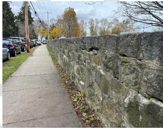
Degraded fieldstone wall along [REDACTED]
