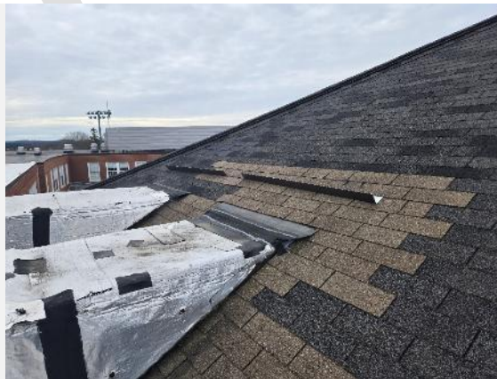
Patched asphalt shingles.
