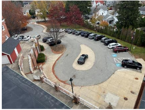
Aerial view of east parking lot.
