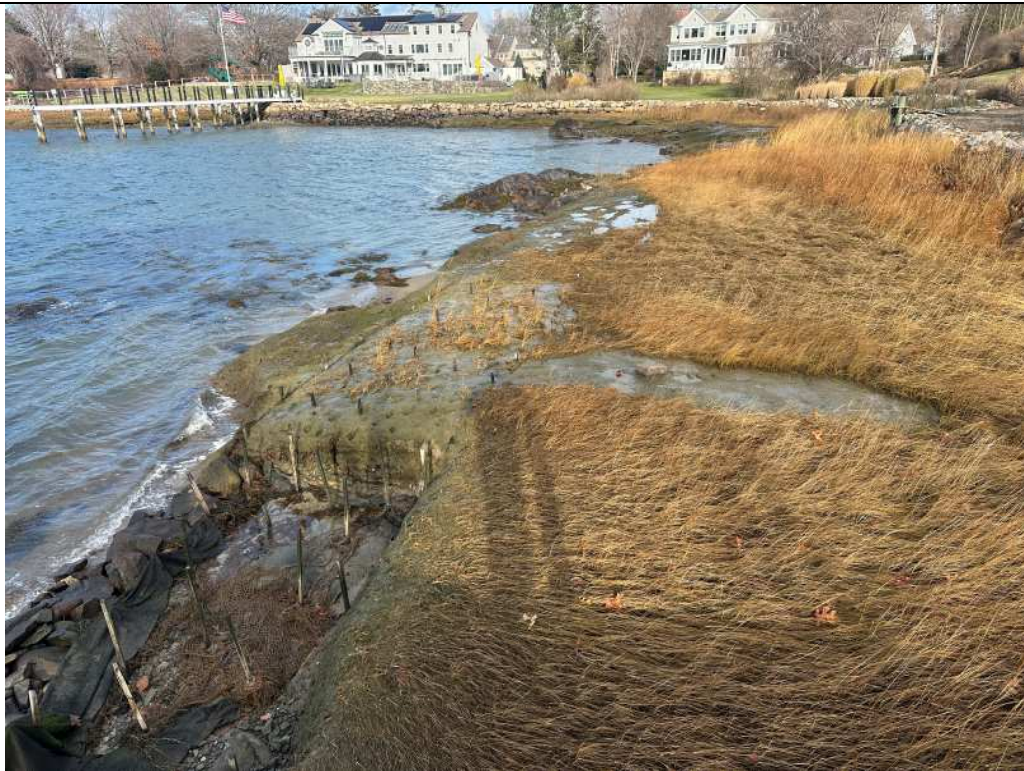
Float damaged area has washed out. Filter fabric and stakes should be removed.
