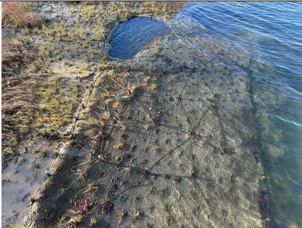
Seaward edge of southern side of salt marsh restoration area. Plantings toward seaward edge too low to thrive.
